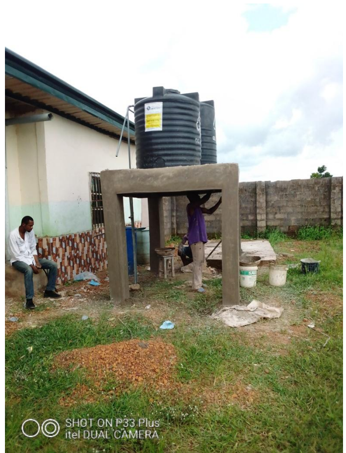
Plastering in Progress.
