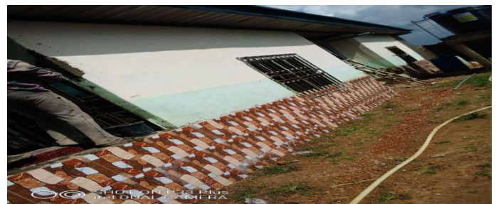
One Side of the building.
