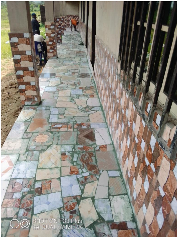
Field side of the Building (At the back).
